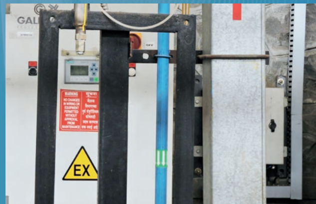
Figure 15: ATEX certified control panel
