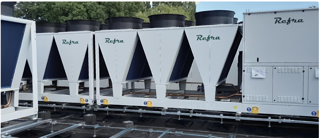
Refra's propane heat pumps being installed at the Solihull district energy network. Photo credit: Absolutely Chilled
