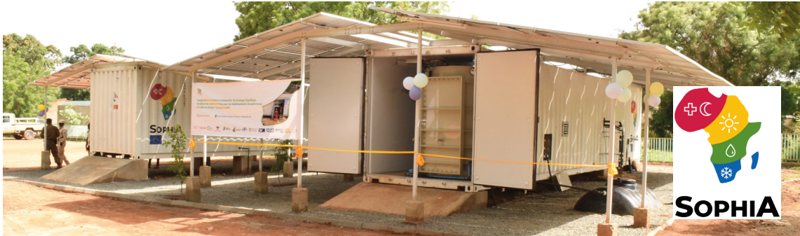
SophiA solar-powered container in Burkina Faso. The facility is equipped with a 1,000l capacity storage for drinking water and a CO 2 /propane cascade system to provide with the refrigeration needs for vaccine storage at +5°C, -30°C and -70°C
