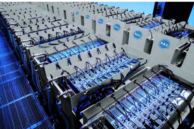
BAC's immersion cooling tanks with CorTex technology. Photo credit: BAC.
