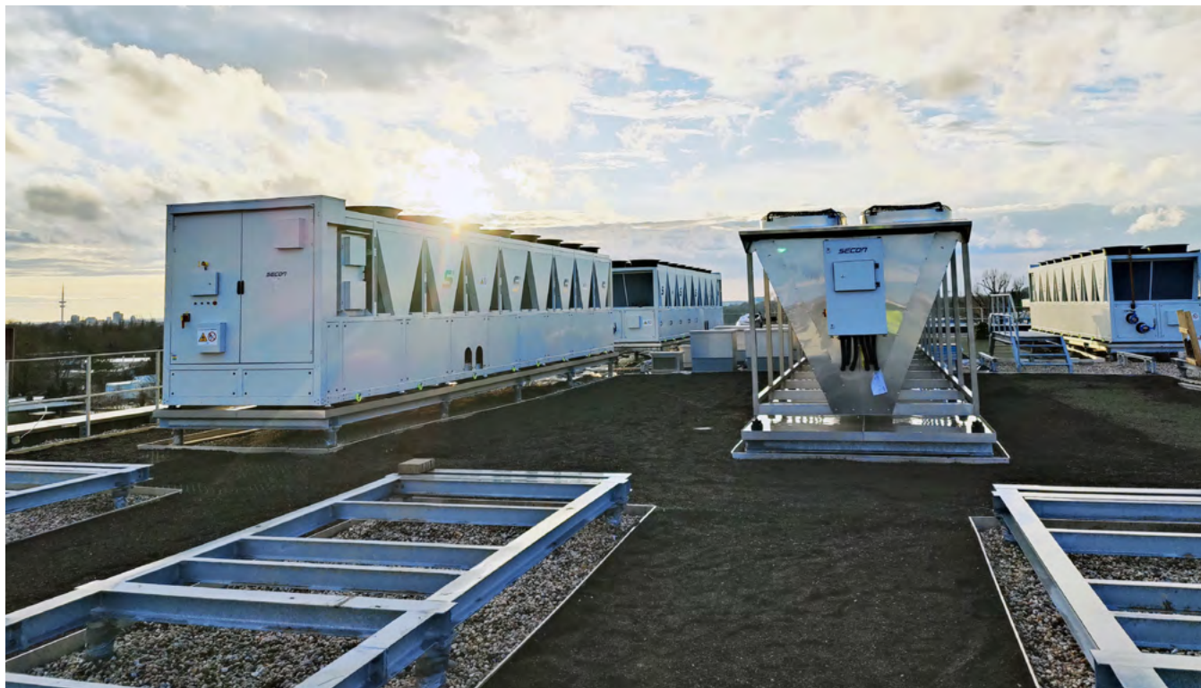
Secon’s propane chillers installed on the roof of HAM01. Photo credit: Secon.
