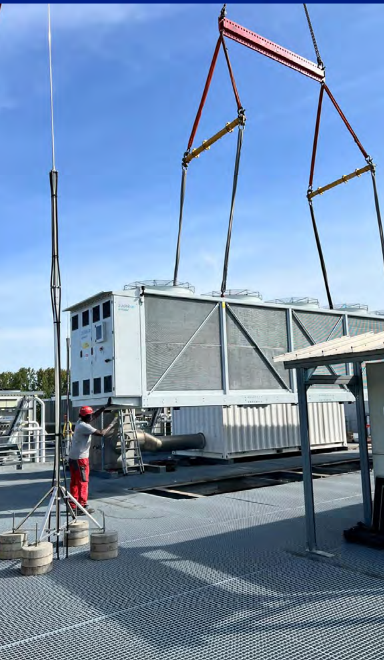
The Airmatik being lifted into place at a data center. Photo credit: Zudek.
