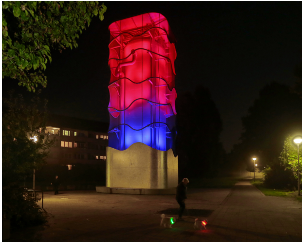
Architectural integration of a district heating water storage tank in Hildesheim. Lighting colour fades from red to blue according to the amount of energy stored in the tank. ©Lighting design
